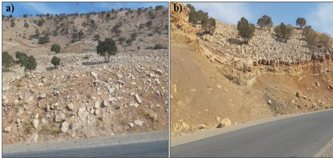
Figure 7: a- Toppled limestone blocks from the Pila Spi Formation over the red clastics of the Gercus Formation (Station No. 6), b- Highly jointed and weathered limestone beds of the Khurmala Formation underlain by the highly weathered clastics of the Kolosh Formation (Near Station No. 7).
